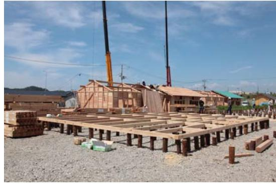
**Emergency temporary housing constructed using a wooden panel system** Kunihiro Ando
